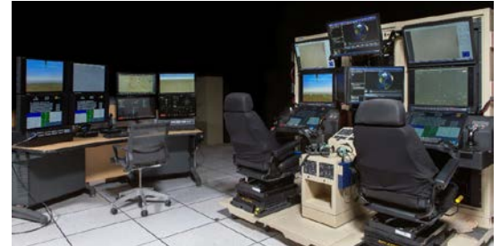
GA-ASI's Flight Test and Training Center in North Dakota is now home to a CAE-built Predator Mission Trainer that will be used to deliver advanced pilot and sensor operator training
